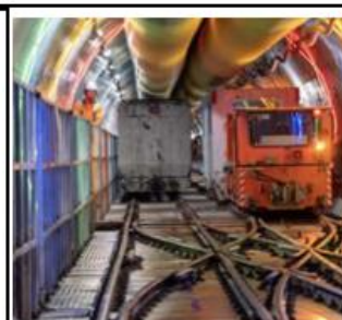
Train in tunnel removes spoil and carries crew to/from work.
