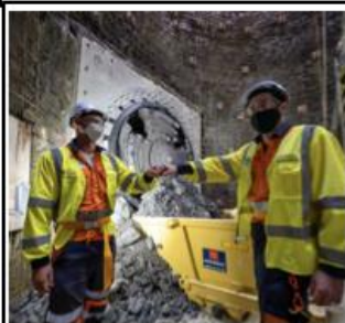
TBM breaking through into shaft
