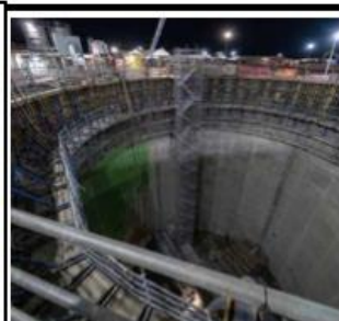
Lining pump station shaft with concrete
