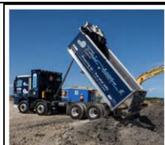
Electric truck carries spoil to Puketutu Is.
