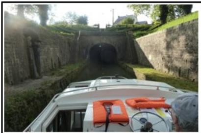
Green light showing tunnel is clear
